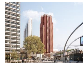
2 Finsgate House Old Street
