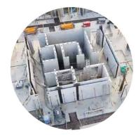
Pre-cast concrete shear / core walls
